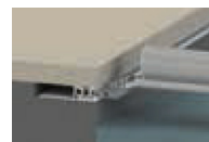
Rail only under the coping
