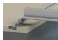
Flush mount rail in the pool surround
